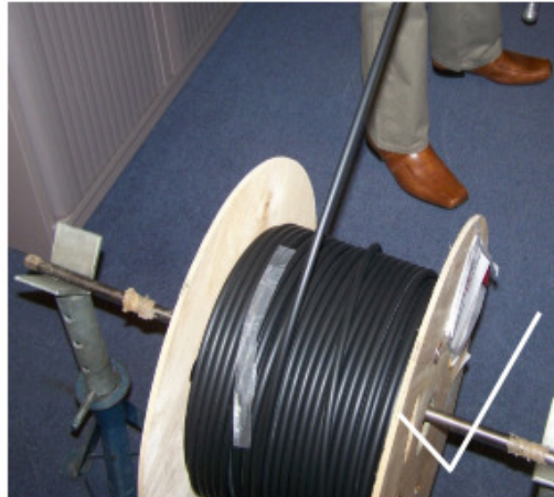
Correct method of de-coiling
